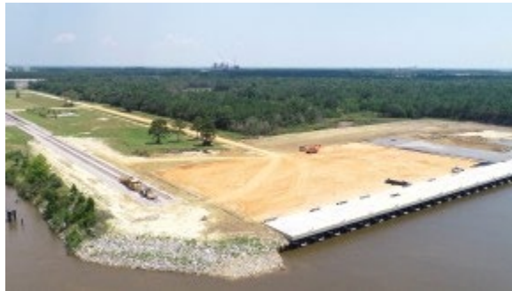
Figure 4 New 600-Foot Barge Dock, Rail and Upland Yard (Source HCPHC)
