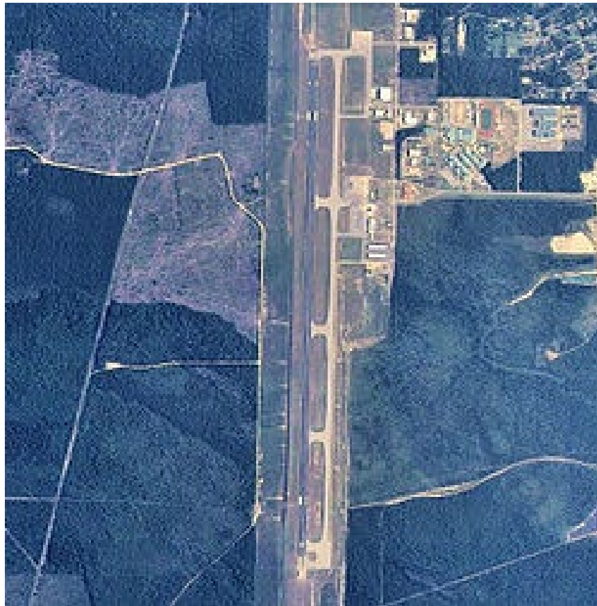
Figure 8 Stennis International Airport (Source: Google Earth)
